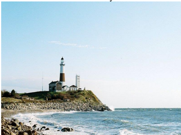
Montauk Point Lighthouse
